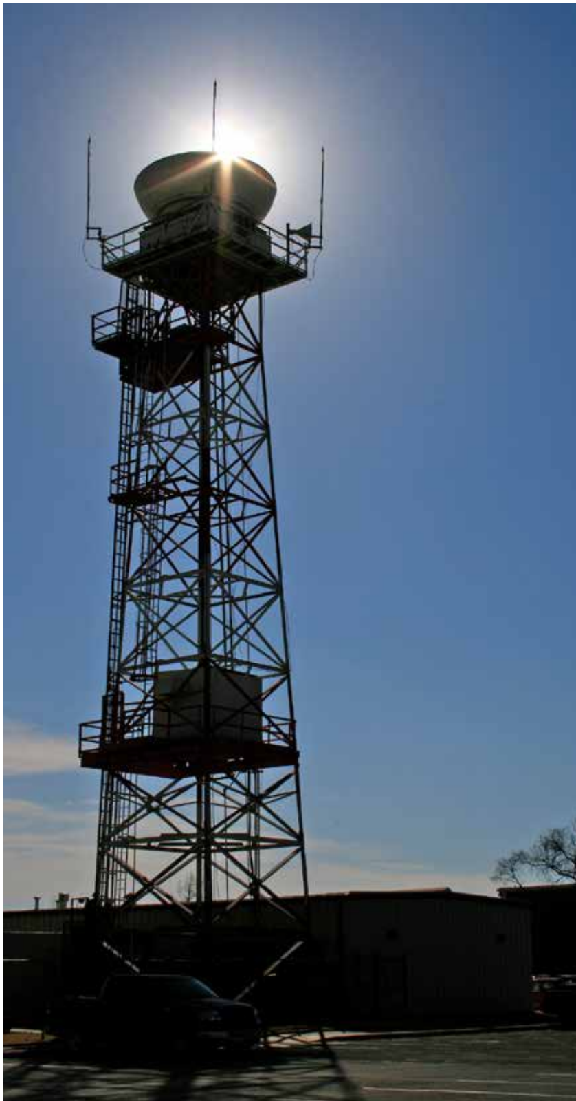
Airport surface detection equipment (ASD-X) gives controllers visibility of all activity on the airfield.
